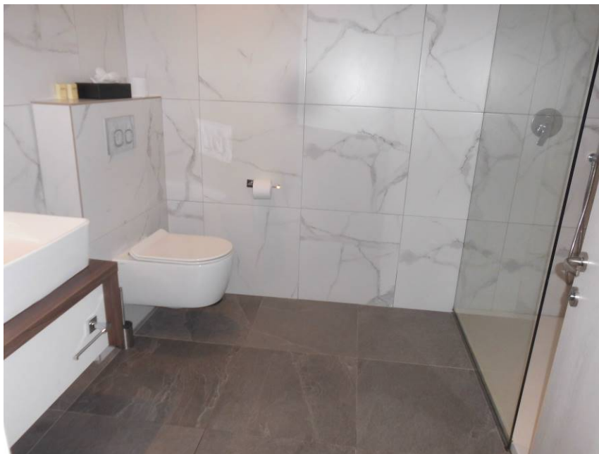
Photo 24: Bathroom facilities to original rooms
