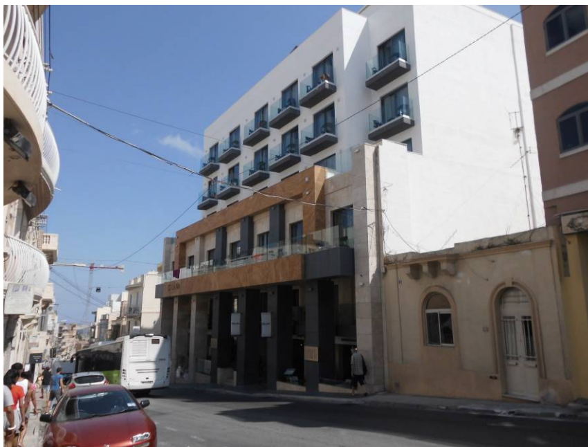
Photo 2: Main facade down the road
