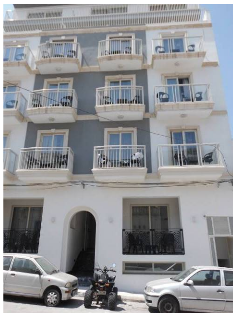
Photo 4: Rear Facade of internal block on Triq Frangisk Zahra
