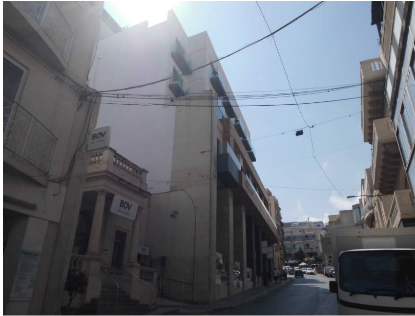
Photo 3: Main facade up the road.
