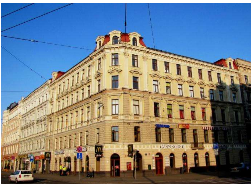
Commercial & office building – Merkela Street, Riga, Latvia
