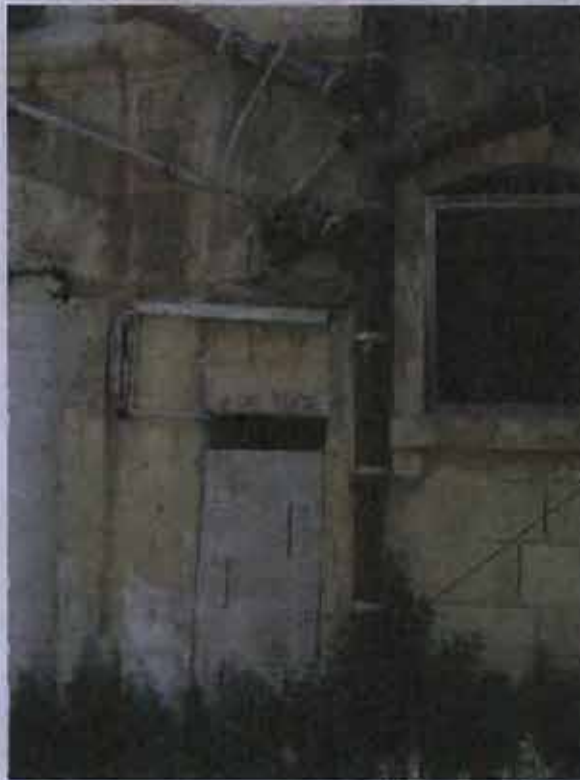
Figure 6: Blocked up wall that is presumed to give access to underground reservoir
